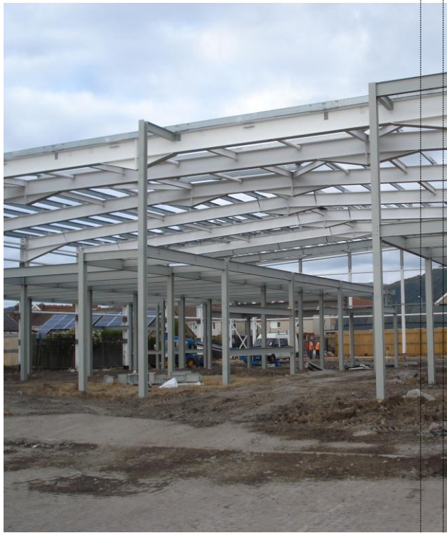
New 1 st floor steelwork.
