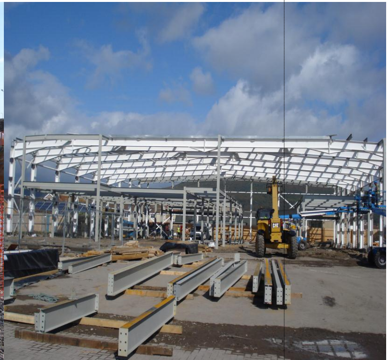
Phase 2 area awaiting steel.
