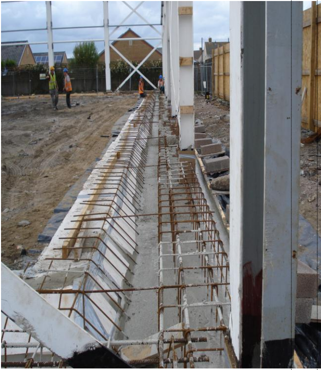
New slab edge detail along GL A.
