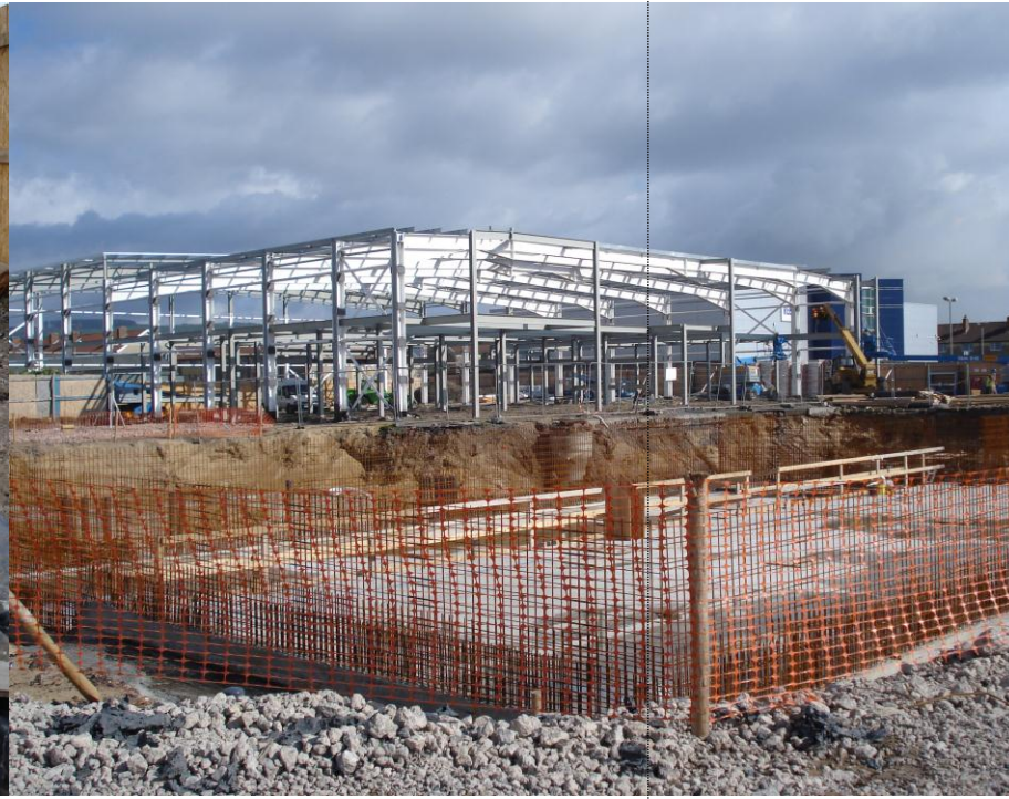
Swimming pool with wall mesh prepared.
